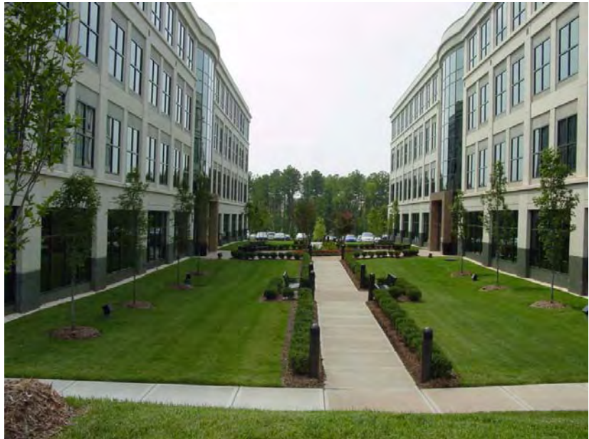
FIGURE 2. A courtyard in a business campus in Raleigh, NC
